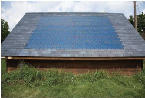
(a) Photovoltaic shingles on a home
