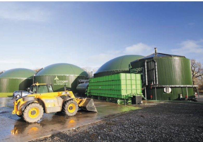
FIGURE 10.6 Anaerobic Bioreactor This bioreactor is used to produce methane from animal manure on a large dairy farm. Ashley Cooper/Getty Images
