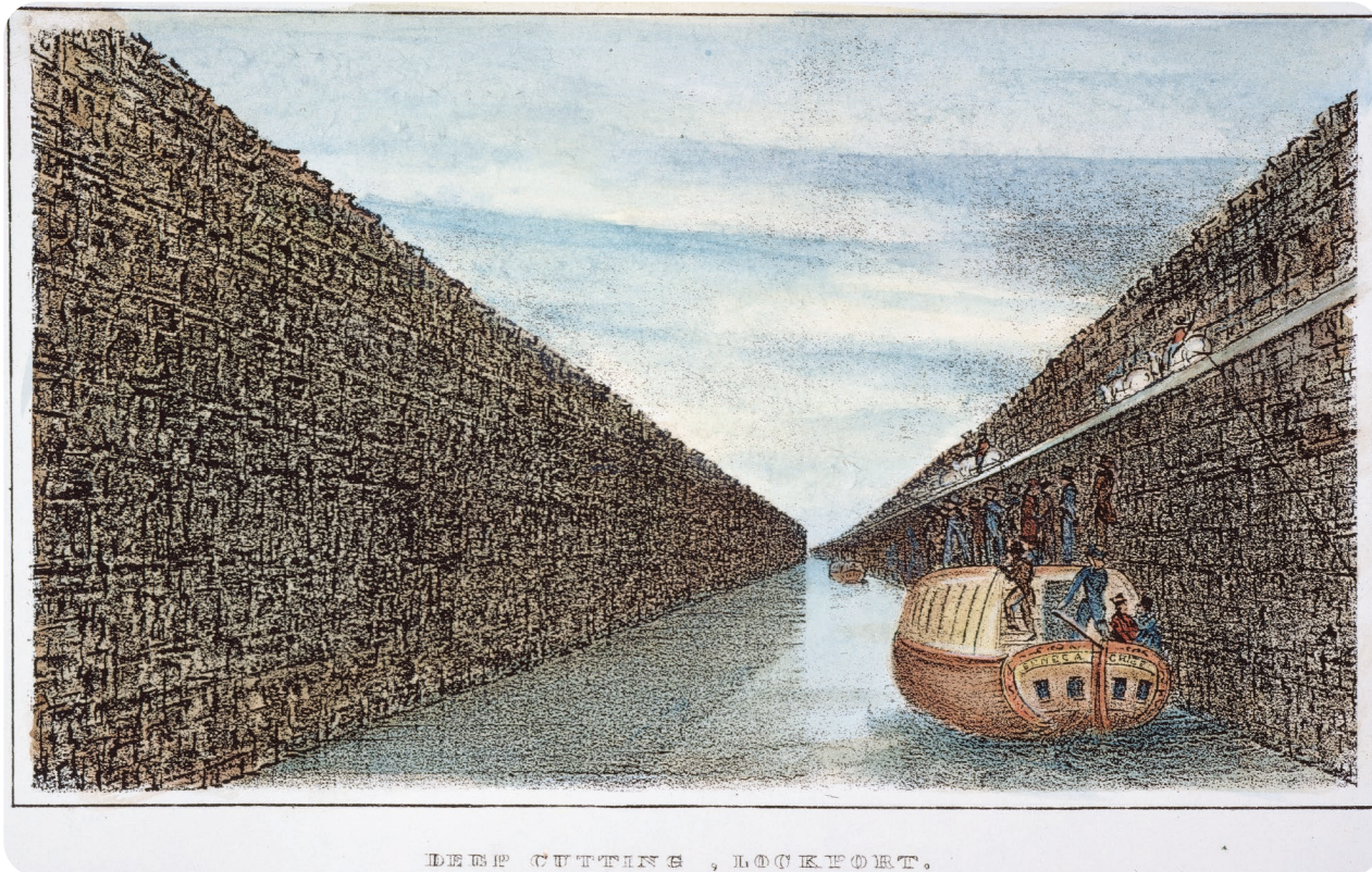
THE ERIE CANAL This lithograph suggests something of the enormous engineering challenges faced by the builders of the Erie Canal. This picture shows a deep cutting at Lockport, New York. The canal was completed in 1825 and connected New York to the Great Lakes via the Hudson River.
