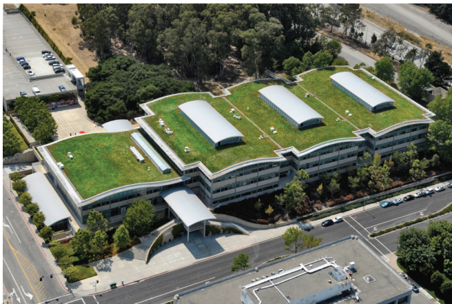
THE GAP CORPORATE HEADQUARTERS BUILDING UTILIZES A GREEN ROOF WITH SOLAR PANELS.
